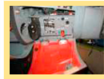
EXTERNAL POWER RECEPTABLE
